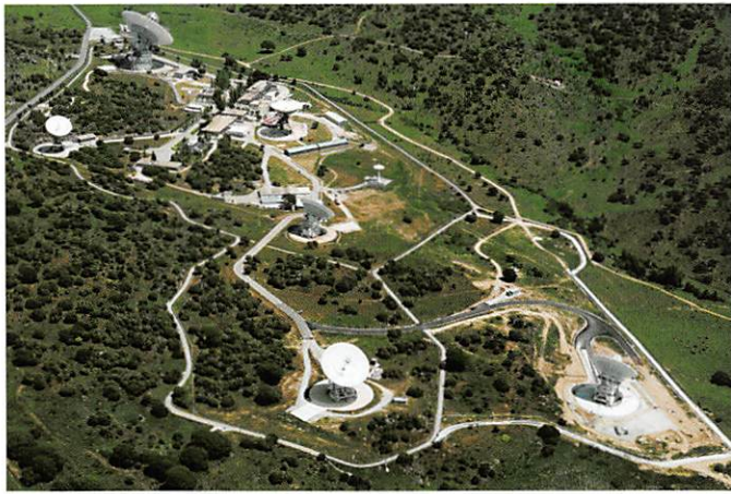
THE MADRID DEEP SPACE COMMUNICATIONS COMPLEX NEAR MADRID, SPAIN. IMAGE COURTESY NASA/JPL-CALTECH
